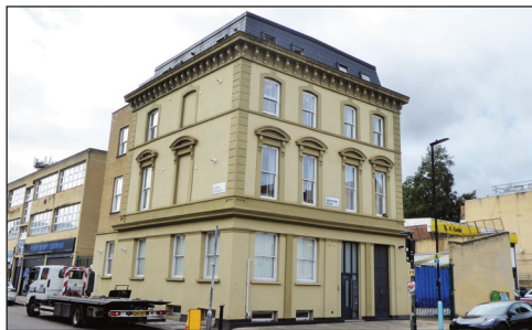
The former Mamelon Tower
